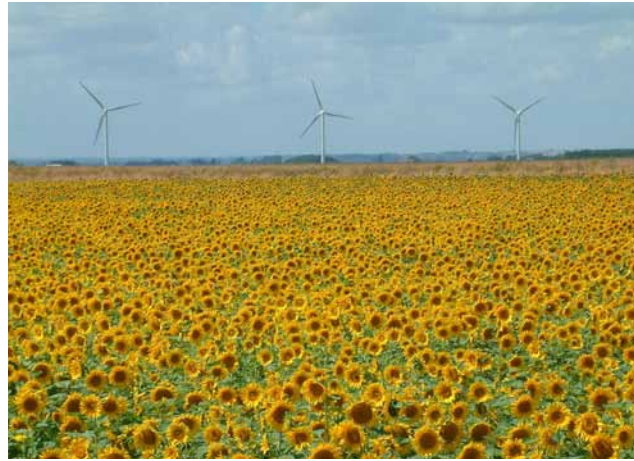
Wind turbines near Depping St Nicholas, Lincolnshire (© Wash Estuary Strategy Group/A Lambert)
